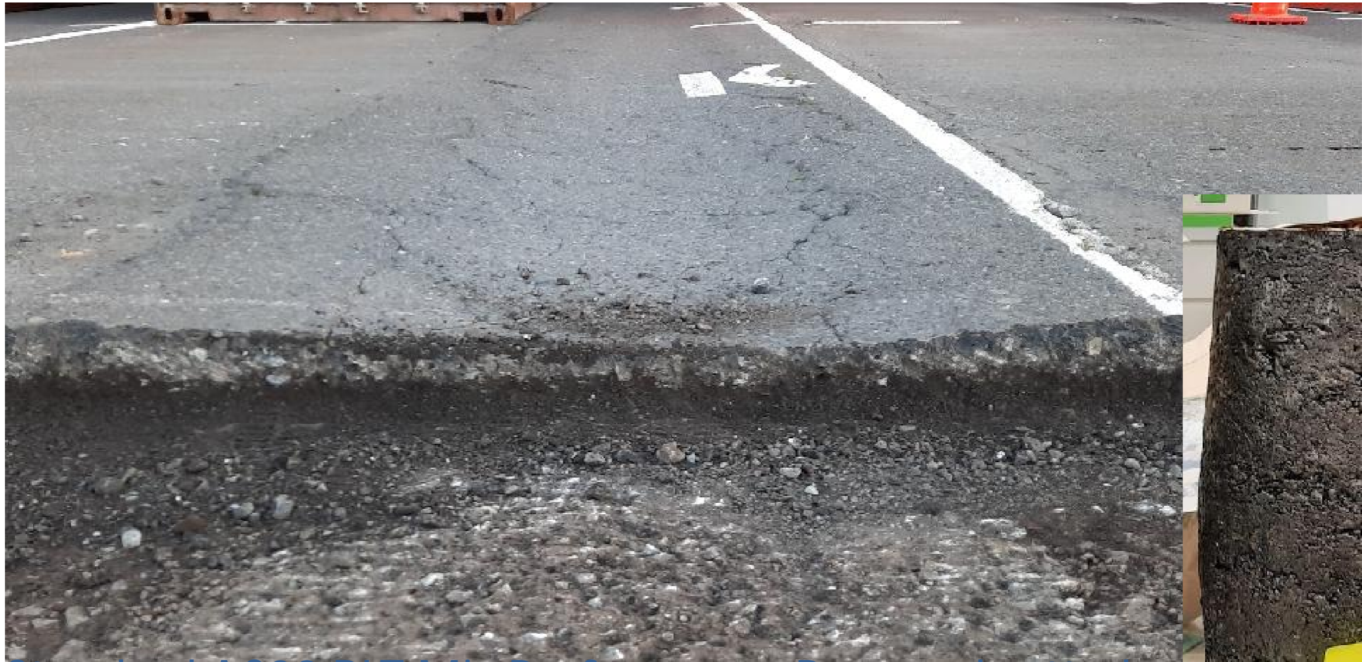
Standard AC28 RLT Mix Performance Poor and rutted (35mm)
